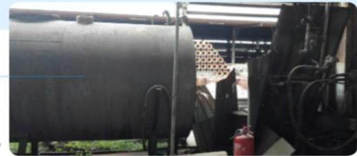
The renewable green energy burning system (fuelled by pulverized palm kernel shell powder) to replace the fuel oil/ diesel burning system.
